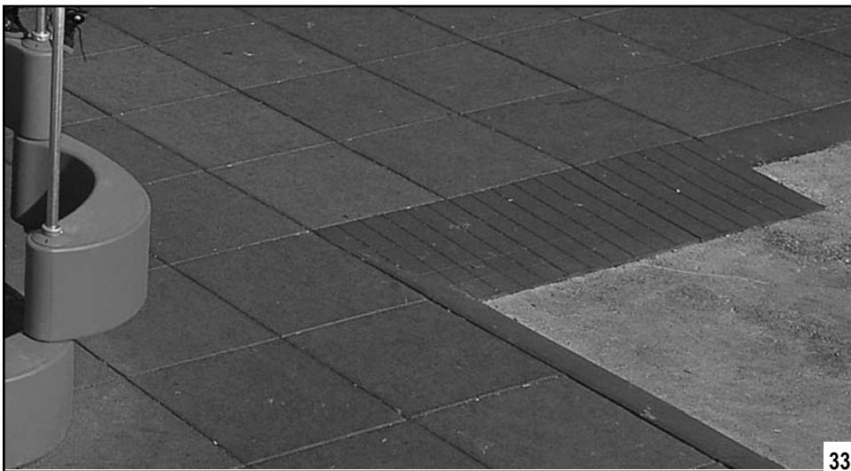
To accommodate a height change along the perimeter of a play area - like these rubber safety tiles placed on an asphalt surface - an allowable 1:12 slope is utilized for the transition at the boundary of the play area.
