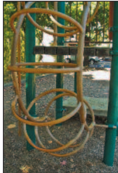
Figure 9: Climber with rigid structural components that DOES NOT meet 5.3.2.1.5
